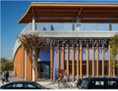
View of Community Center entrance, showing wood louvers and rooftop canopy, phenolic panel rainscreen and custom stainless steel railings - Photo Credit: © Paul Warchol
