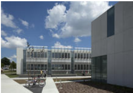
Courtyard View to North - Photo Credit: Assassi
