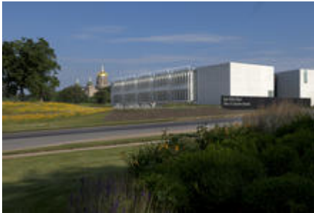
IUB-OCA Building - Photo Credit: Assassi
