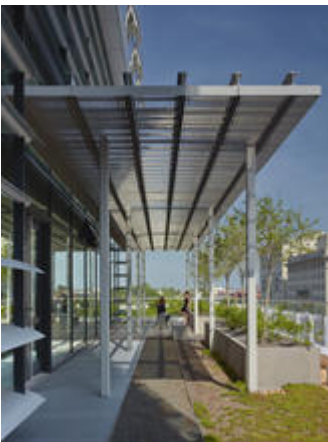
Roof terraces provide users with access to fresh air and collect rainwater runoff for remediation and reuse. - Photo Credit: Brad Feinknopf
