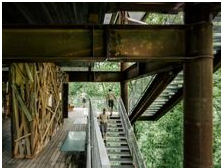
Dynamic circulation is integral to the treehouse experience and recalls the fascination of childhood play. - Photo Credit: Photography by Joe Fletcher
