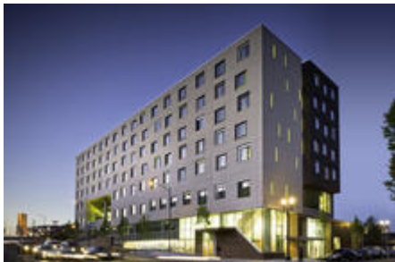
Bud Clark Commons; Dusk view from SW. - Photo Credit: Christian Columbres Photography
