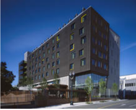
View of Bud Clark Commons from the northeast, including custom entrance gate that leads to public courtyard for the homeless seeking services and shelter. - Photo Credit: Sally Schoolmaster
