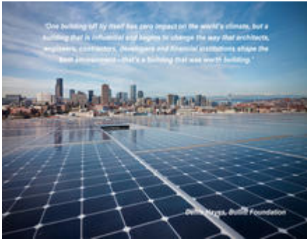
PV array - Photo Credit: Nic Lehoux
