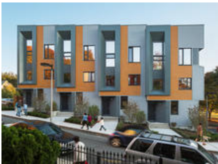
View from Highland Street - Photo Credit: Sam Oberter
