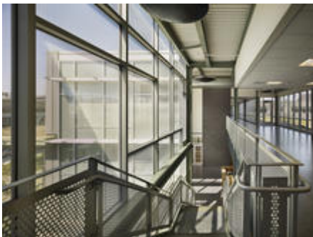
Recycled content steel, masonry, glass and drywall from PA - Photo Credit: Barry
