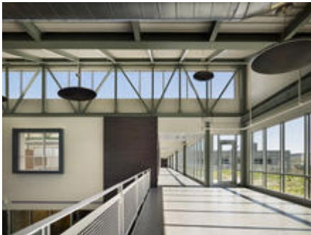
Daylighting with clerestories, skylights and borrowed light - Photo Credit: Barry Halkin, Halkin Photography
